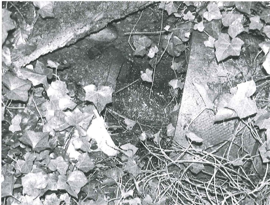
Photograph 3. View of poor / damaged storm drain connection.
