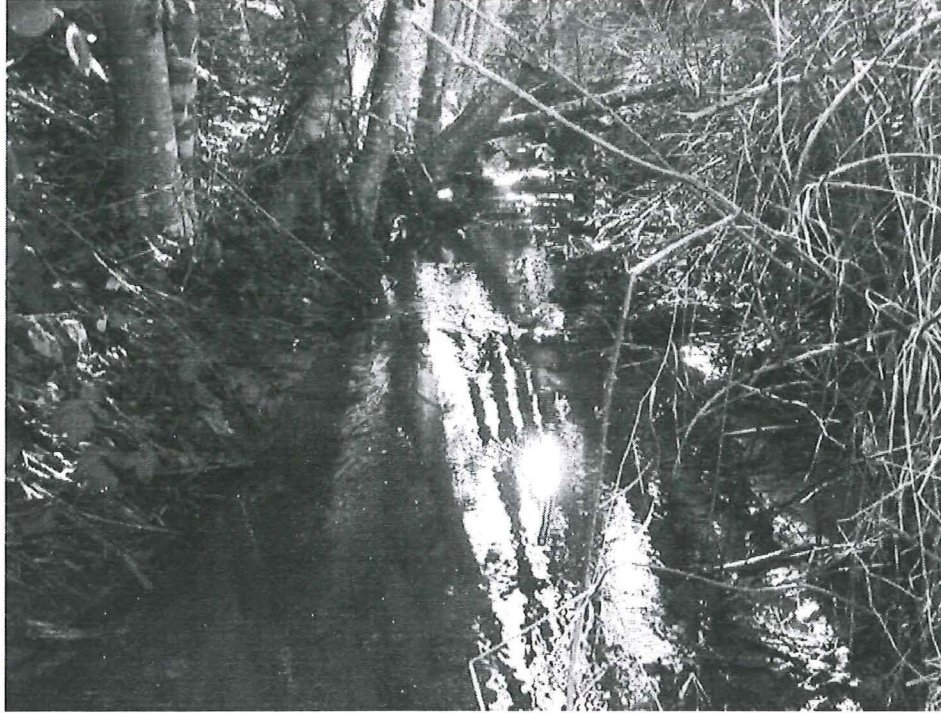
Photograph 4. View downstream from the culvert under Extension Road.
